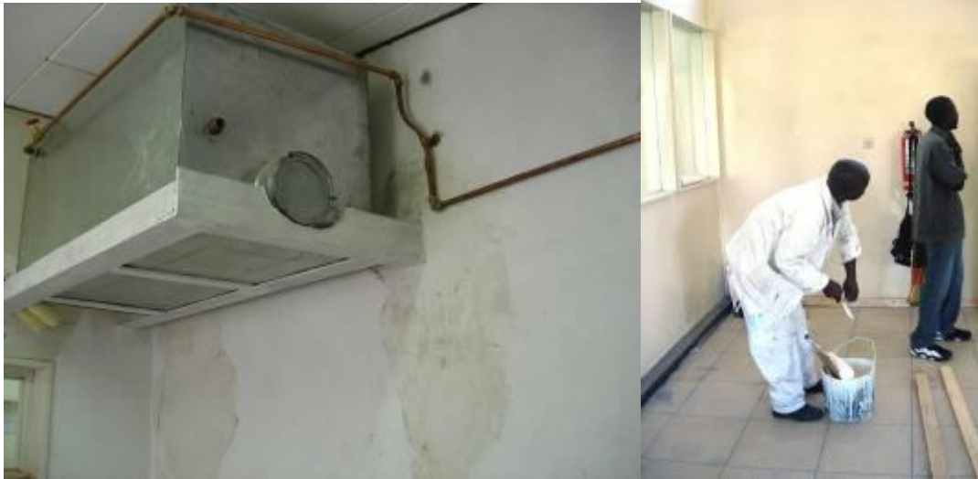
(left) Hot water geyser donated by ZimHealth and (right) Painters and Carpenters at work
